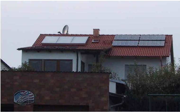
Fig. 12.1. Typical roof-mounted installation of a solar-thermal and PV system. (Source: Mayer, private photograph)
