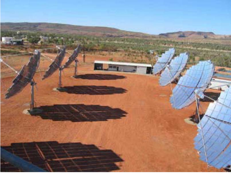
Fig. 2.10. 190 kWp power station by Solar Systems [27]
