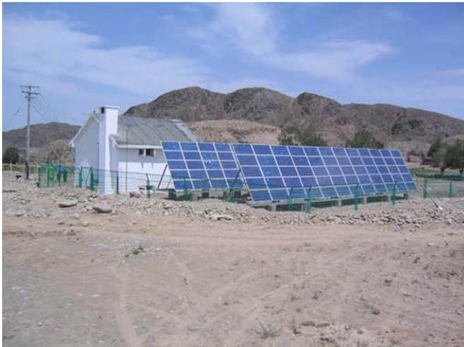
Fig. 12.4. PV generator for a village electricity supply. (Source: SMA)
