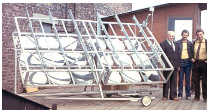
Fig. 8.19. Solar PV installation with AlGaAs/GaAs solar cells and parabolic mirrors, 1981 [118]. In photo: Alferov ( on the right ), Rumyantsev ( in the center ) and Tuchkevich, former director of Ioffe Institute
